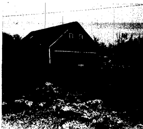
SMOLDERING RUINS mark the site of the Clark Smith, Jr. barn south of Laurel following Sunday's fire. The barn, haystacks and hogs burned. A ruined coaster wagon stands overturned in the debris. Smoke from the still-smoldering debris shows haze like in front of outbuildings.
